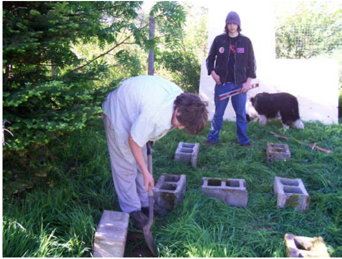
Levelling down more blocks....
