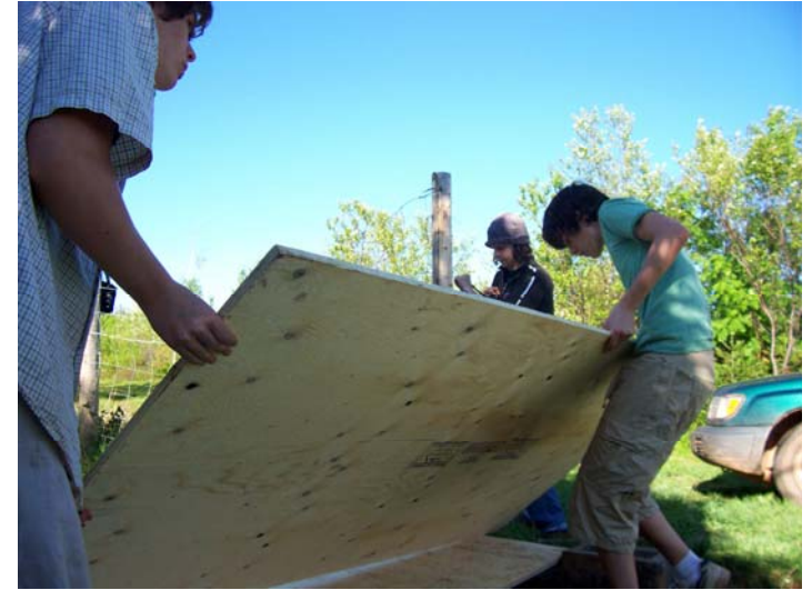
The plywood floor goes down...
