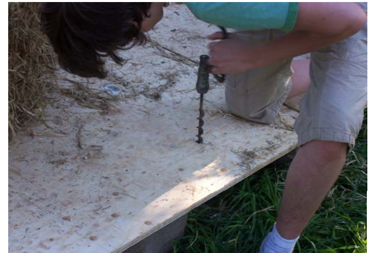
...and is drilled the old fashioned way.
